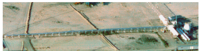
Fig. 12. Overhead view of Spill Test Facility at NTS, showing two 100 m 3 cryogenic tanks, two 150 m long spill lines, and supporting equipment.
